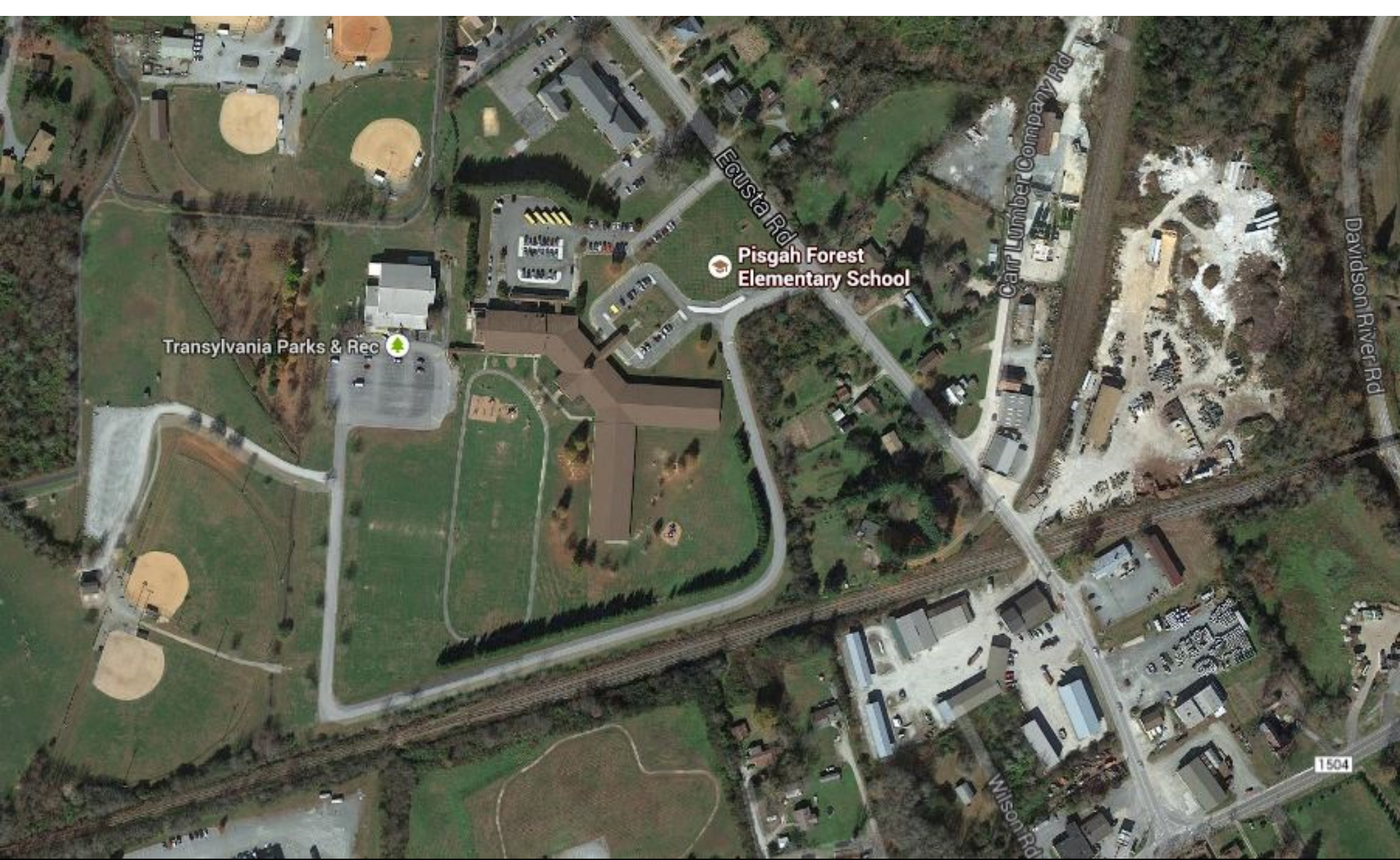
Pisgah Forest Elementary School
